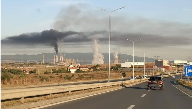
Figure 3: Power Plant in Obliq Source: ATRC, KOSOVO
