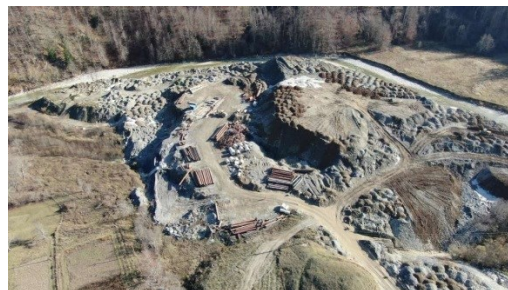
Figure 18- Source: Unesco report: highway construction damaged tara river
